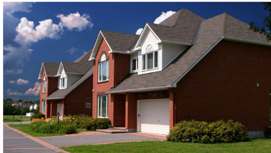
Figure 1 CCHT twin houses (www.ccht-cctr.gc.ca)
